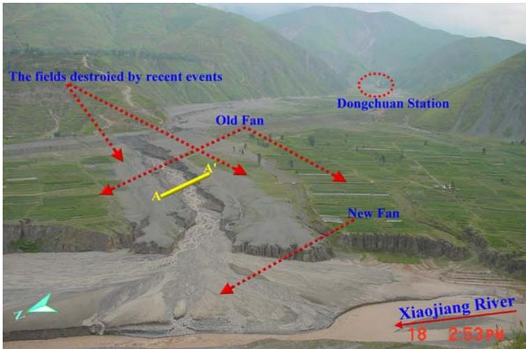
**Fig. 2** Huge debris-flow fan in the confluence of Jiangjia Ravine with Xiaojiang River (face to upstream). Debris flows on August 20th, 2001 in Jiangjia made a serious damage to the crops planted in the alluvial fan by local farmers. The channel width at section A–A' is about 45.0 m
