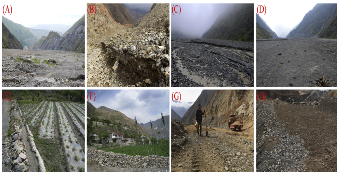
Fig. 4. Original conditions and consolidation of the debris flow waste-shoal land (DFWSL) in the study area, with uneven micro-landforms, including (A, D) ridges, (B) gravel, and (C) trenches as well as (E, F) large stones for terraces. (G) The DFWSL was flattened, and (H) mature soil from nearby areas was moved to increase the composition of loamy soil.
