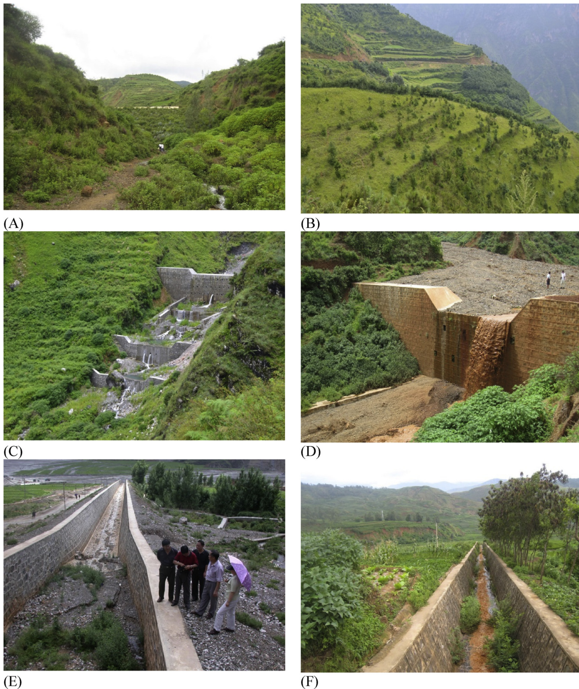
Fig. 9. Various measures for ecological preservation: (A, B) slope ecological protection measures; (C, D) check dam; and (E, F) drainage groove.
