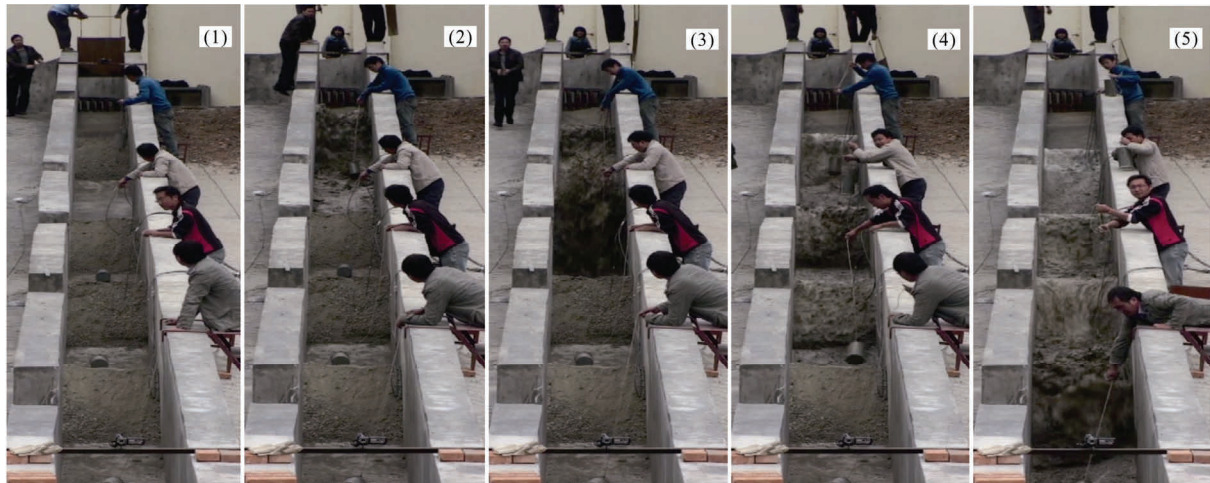
a. Complete blockage
