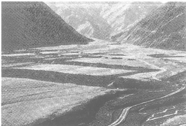
Photo 6A. The deposition size with earth-dams designed to catch the mudflow mass.
