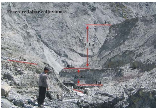
Fig. 9 Site photograph showing fast cutting and severe erosion in Menqian ravine, position (1,660E, 1,280N)
